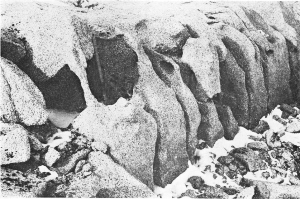
Fig. 7. Thin rock bridges across a complex erosion cavity in granodiorite (E.4076). The hammer shaft is graduated at 5 cm. intervals.
