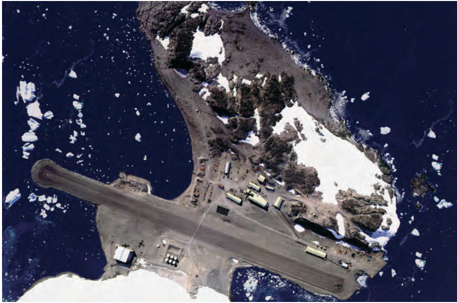
Left: The long, crushed gravel, runway at Rothera is clearly visible as is the hangar and the fuel storage tanks (bottom left). Discernable outside the hangar are two Twin Otters with a third on the right-hand end of the runway preparing for take-off. (BAS / NERC ©)
